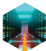
Telecom & Data Centers
