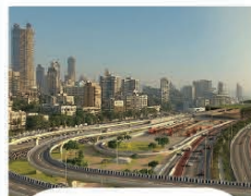
MUMBAI COASTAL ROAD MEGA PROJECT
