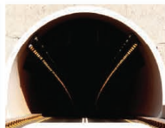
AIROLI-KATAI NAKA TUNNEL
