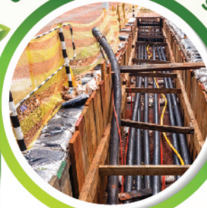
Underground Cabling
