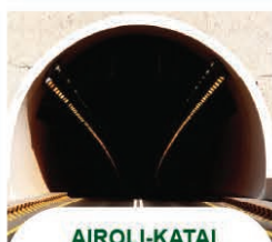
AIROLI-KATAI NAKA TUNNEL
