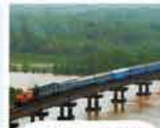
KONKAN RAILWAY PROJECT
