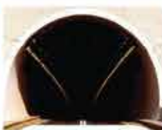
AIROLI-KATAI NAKA TUNNEL
