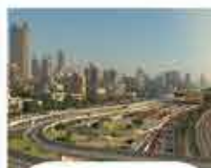
MUMBAI COASTAL ROAD MEGA PROJECT
