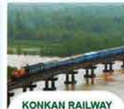
KONKAN RAILWAY PROJECT
