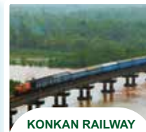
KONKAN RAILWAY PROJECT
