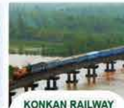
KONKAN RAILWAY PROJECT
