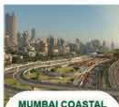
MUMBAI COASTAL ROAD MEGA PROJECT
