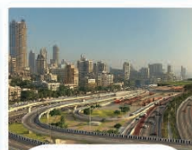
MUMBAI COASTAL ROAD MEGA PROJECT
