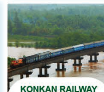
KONKAN RAILWAY PROJECT
